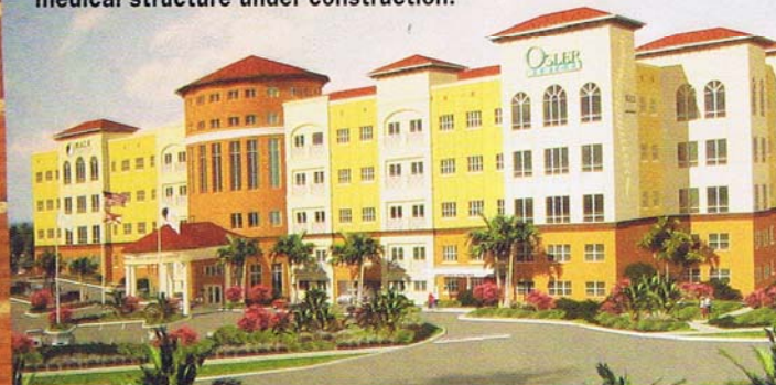
DAVE MENZEL , President of MAI Design Build, with a rendering of the Crane Creek Medical Center. Below, the 210,000 square foot medical structure under construction.
